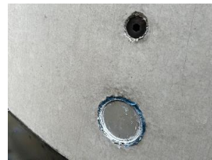
(b) Installation of pore water pressure gauges and soil pressure gauges
