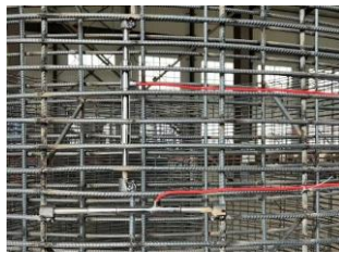
(a) Reinforcement gauge installation
